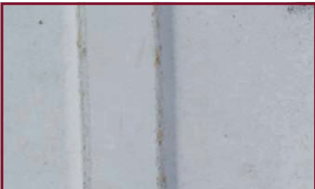
Panel bend corrosion after 21 years
